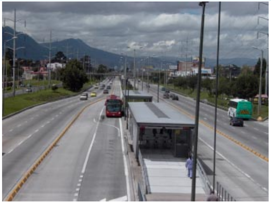
In the central aisle of this expressway, Bogotá's TransMilenio has modular passenger stations divided into local and express units serving the corresponding vehicles, which travel on double exclusive lanes. Pedestrian bridges provide access to these stations.
